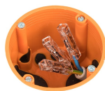
Extending short wires.
